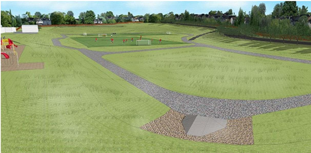
Figure 1. A Dry Pond design in Calgary<sup>6</sup>
