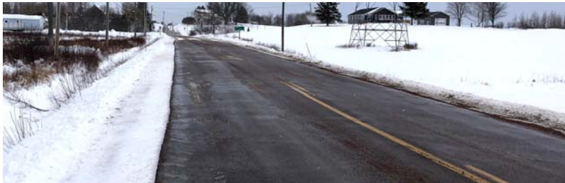
Photo 1 – Pond Shore Road Near Town Limits
