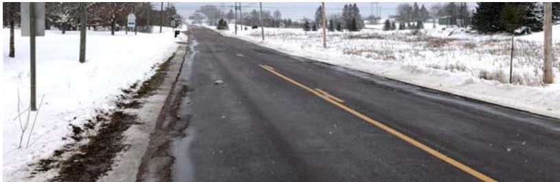
Photo 2 – Pond Shore Road Near Mount View Road / Station Road
